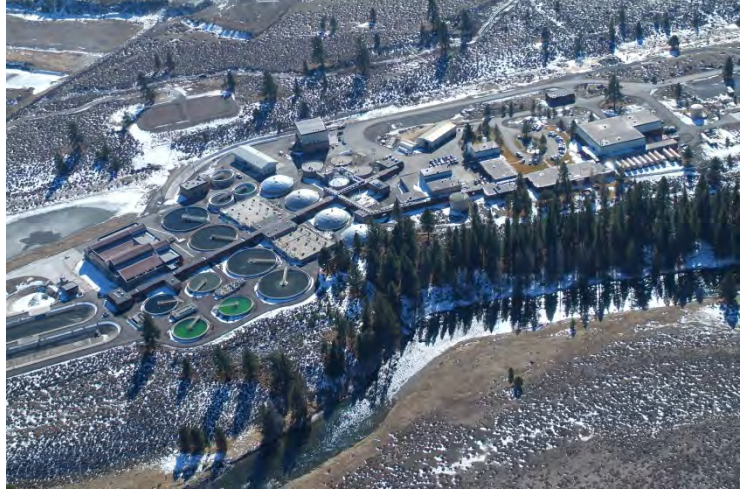
Aerial photo of T-TSA Wastewater Reclamation Plant
